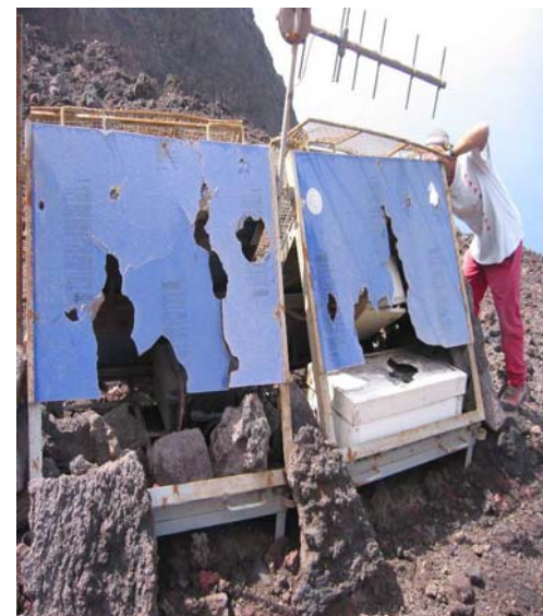
Concrete reference station destroyed by the volcano.
