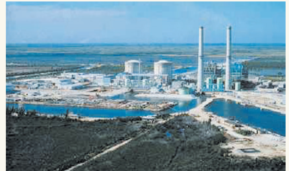
High-definition surveying is used heavily in the power plant industry. Image courtesy: Framatome ANP
