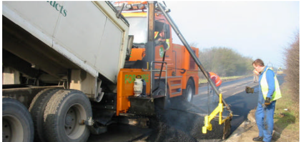
The flexible Sidewinder can place material on either side of the machine
