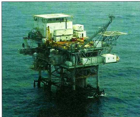
Chevron's EI 252 I platform, with a capacity to handle 20,000 bo/d, lies 83 miles offshore Louisiana (Fig. 1).
