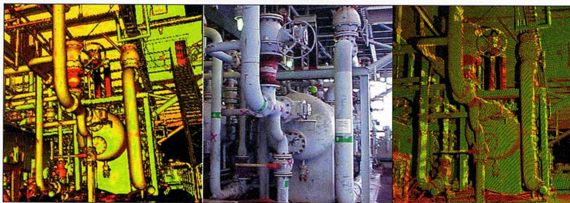
A comparison of images shows the shrink-wrap laser scan on the left, a digital photo in the middle, and the laser scan on the right (Fig. 4).
