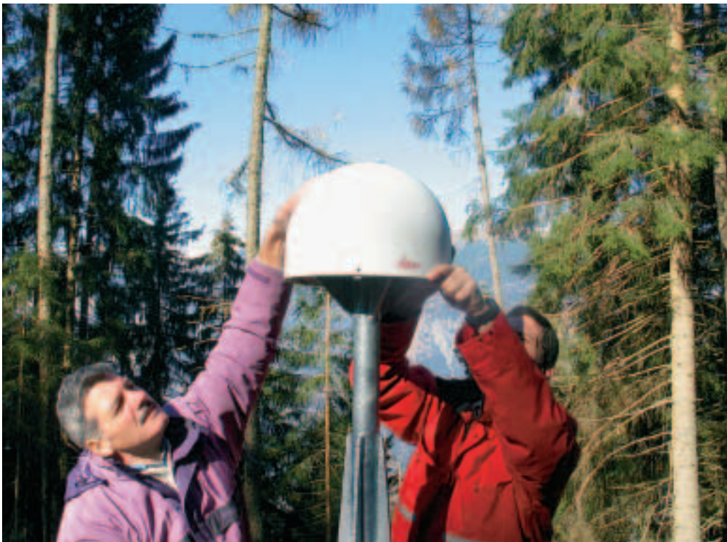
(Below): Erwin Truttmann (Rost) and Christoph Kandler, Manager of Weiser-Kandler, installing the GPS antennas. Despite the dense vegetation that formed significant obstructions for GPS signals, Leica SmartTrack technology provided the high accuracy data needed for monitoring applications.
