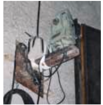
Leica TCR1105 total stations are mounted high on the walls where they undertake surveying and monitoring work
