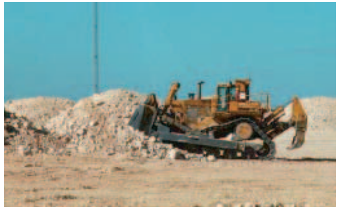
(Above): Dozer 2000 - the position of the earth moving machine relative to the desired "design" surface is displayed to the Dozer operator
