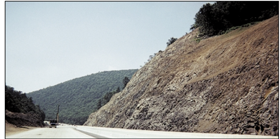
Rock wall adjacent to SR 322 at Mt. Pleasant, PA.
